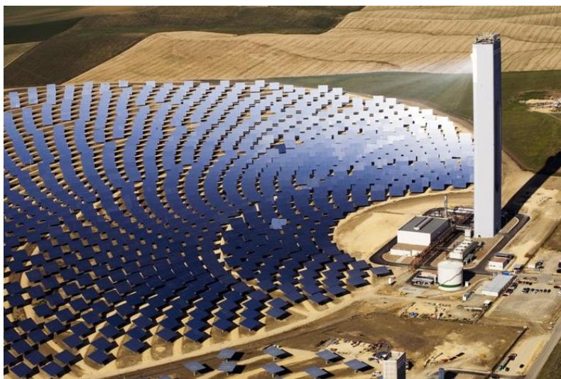
Figure 2: Solar Concentrator Thermal Power Plant [6]
